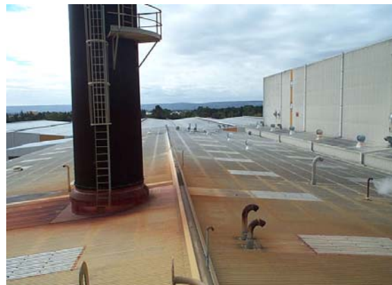
Water collection from roofs
