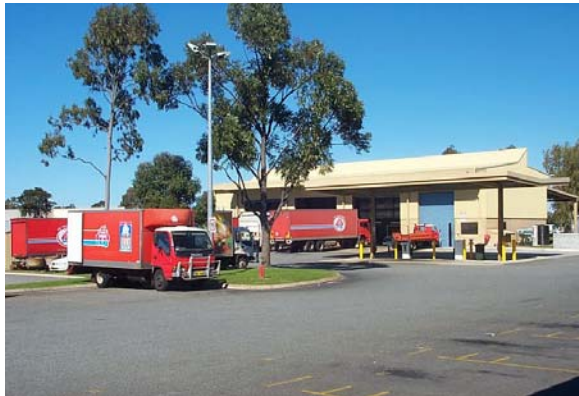
Vehicle maintenance workshop
